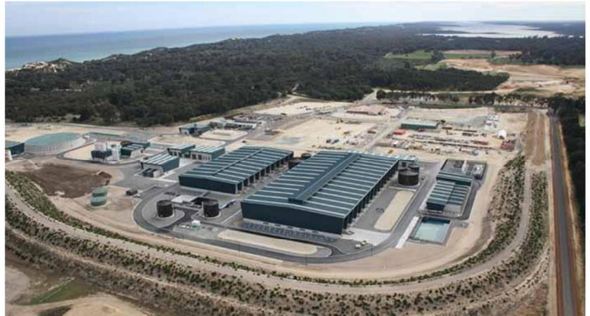
The project included the laying of a 30 kilometres of 1.3m (51") pipeline to the South West Integrated System via ultimately two 32ML storage tanks near Harvey. The total cost of the project is \$1.085 billion, and comprises seawater intake tunnels, seawater pumping station, Filtration, Microfiltration, Reverse Osmosis, Chemical dosing, Storage and Transfer systems.
